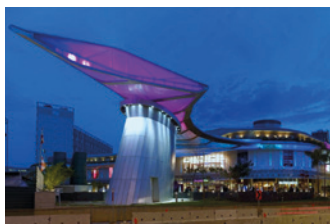
Changi City Point Shopping Mall Сингапур
